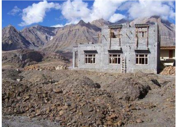
The nearly completed assembly hall
