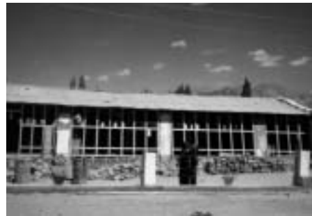
Ladakh - solar heating for weaving workshop
