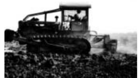
Clearing land in South India
