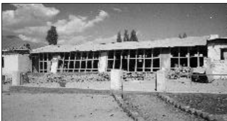
Choglamsar Weaving Shed with new Solar Wall
